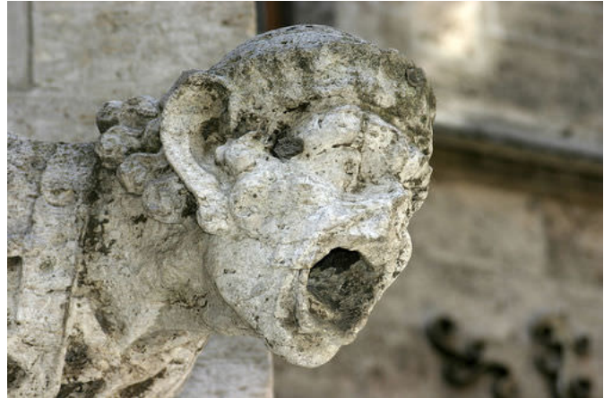
Figure 2. A gargoyles that has been damaged by acid rain.
