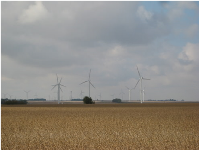
Figure 5. Twin Groves Wind Farm, Illinois Wind power is becoming a more popular source of energy in the United States. Source: Office of Sustainability, UIC
