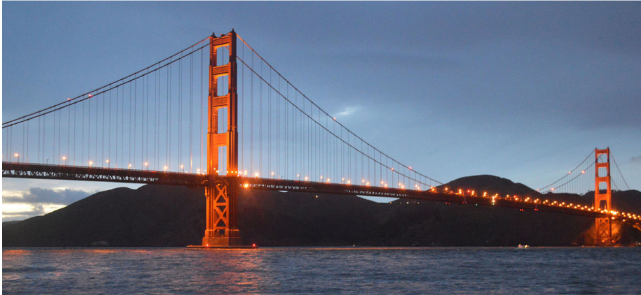
Figure 5.1 The Golden Gate Bridge, one of the greatest works of modern engineering, was the longest suspension bridge in the world in the year it opened, 1937. It is still among the 10 longest suspension bridges as of this writing. In designing and building a bridge, what physics must we consider? What forces act on the bridge? What forces keep the bridge from falling? How do the towers, cables, and ground interact to maintain stability?
