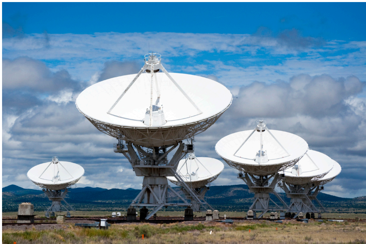
Figure 2.1 The Karl G. Jansky Very Large Array, located in Socorro, New Mexico, consists of a large number of radio telescopes that can collect radio waves and collate them as if they were gathering waves over a huge area with no gaps in coverage. (credit: modification of work by CGP Grey, Wikimedia Commons)
